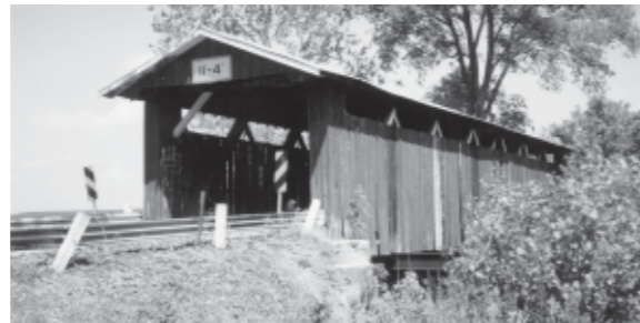
Ballard Road Bridge
