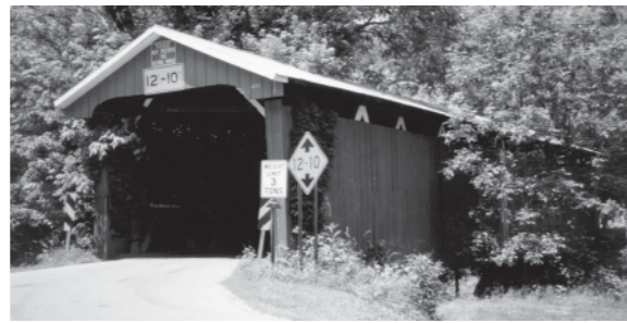
Stephenson Road Bridge
