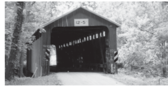
Charleton Mill Road Bridge
