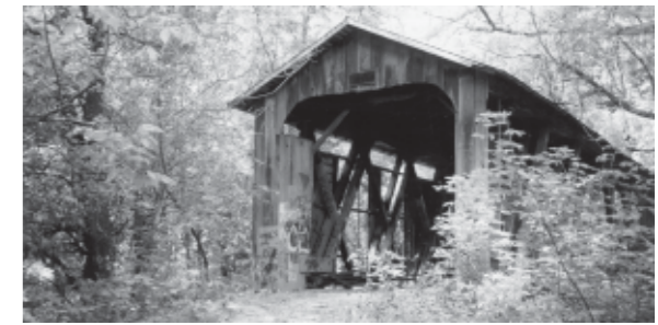
Glen Helen Bridge
