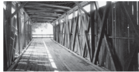
Engle Mill Road Bridge
